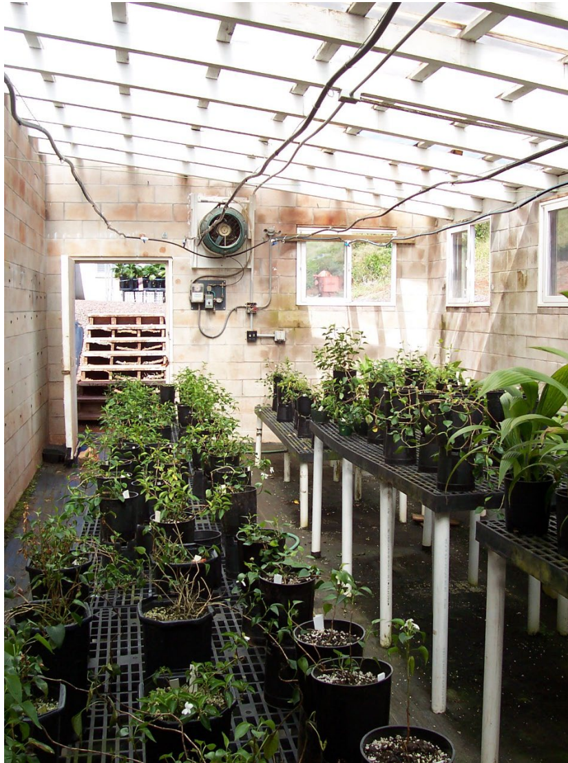
Figure 1.13. A semi-underground growing area used during ANRPO's earlier years at Pahole. Note the intake fan at the front of the structure to encourage air circulation.
