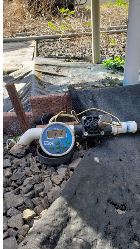
Figure 1.12a and 1.12b. Wiring scheme for the ANRPO main greenhouse controller at Schofield Barracks with AC power, a rain sensor and 48 irrigation zones (1.12a). An example of a battery operated timer (Hunter Node 100) and a 9v solenoid irrigating an outside table at ANRPO’s East Baseyard (1.12b).
