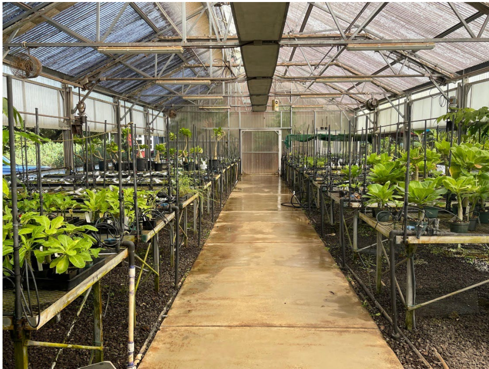
Figure 1.15a and 1.15b. A polycarbonate panel greenhouse used by Pohakuloa Training Area Natural Resources Office (1.15a). Note the motorized vents at the sides and peak of the greenhouse to encourage air circulation. A similar polycarbonate paneled greenhouse is used at the National Tropical Botanical Garden, complete with lights, fans and side and peak vents (1.15b, photo courtesy of Rhian Campbell).
