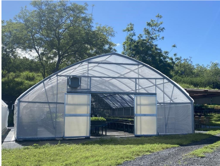
Figure 1.04. Example of a gothic arch greenhouse with polyethylene covering and a solar ventilation fan (Future Forests Nursery Greenhouse, photo courtesy of Jill Wagner).
