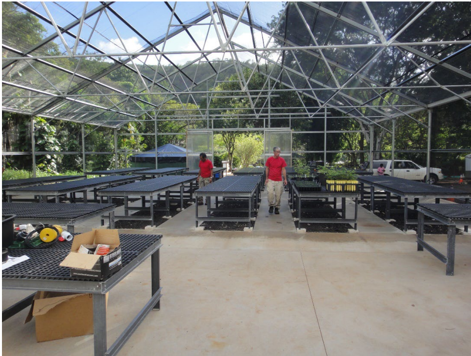
Figure 1.16. A hybrid floor design at Waimea Botanical Garden using concrete to provide level walking paths and gravel beneath the benches to encourage good drainage in the nursery.
