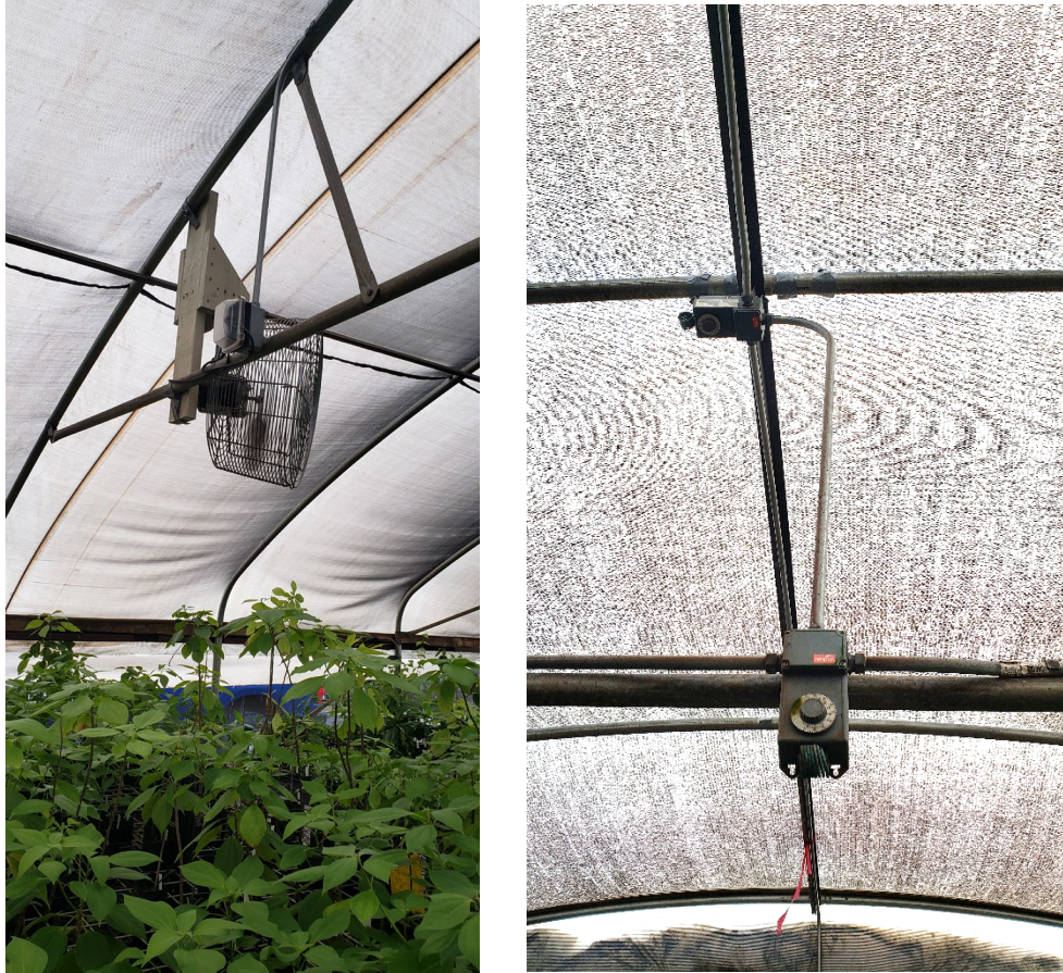
Figure 1.14a and 1.14b. A single circulator fan connected to a GFCI outlet in the ANRPO greenhouse at Schofield Barracks (1.14a). Note the fan's orientation at an angle to circulate air in a circular pattern. Temperature controllers at the peak of the greenhouse and at crop height control when fans turn on/off (1.14b). A ladder is required to change the settings.
